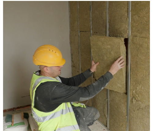
Internal wall insulation
