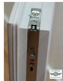
Multi-point locking mechanism (Source: Sashed)
