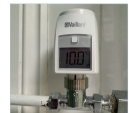
Heating controls Install smart radiator valves to control temperature in individual rooms.
