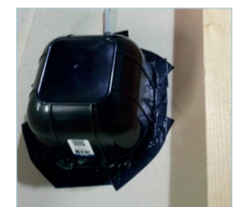
Thermal covers installed in lofts over the back of LED downlights prevent heat escaping.
