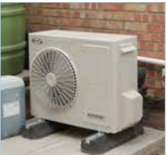
Air source heat pumps collect heat from the outside air and transfer it to your heating and hot water systems.
