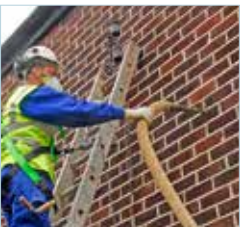
Cavity wall insulation. Polystyrene beads in resin are blown into the wall cavity through drilled holes.
