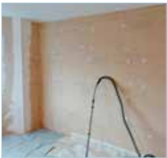
Internal insulation Woodfibre boards applied to inside of external walls and covered with lime plaster.
