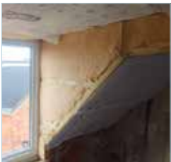
Room-in-roof Insulate internally with wood fibre to keep them warm in winter and cool in summer.
