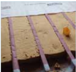
Insulate timber floors. Drape membrane between floor joists and lay mineral wool snugly in between.
