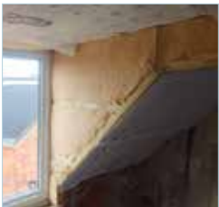
Room-in-roof insulation Insulate roof rooms internally with wood fibre to keep warm in winter and cool in summer.
