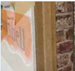
External wall insulation boards covered with a special render applied to the outside of the house.
