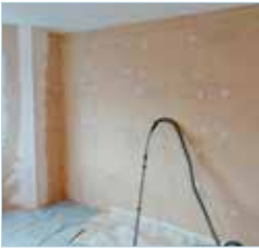
Internal wall insulation Wood fibre boards are applied to the inside of external walls and covered with lime plaster.
