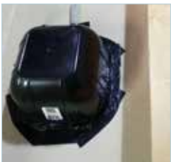
Thermal covers installed in lofts over the back of LED downlights prevent heat escaping.
