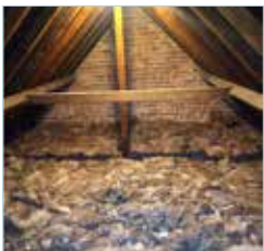
Loft insulation Extra layers of insulation (up to 300mm) are rolled out between and over the joists in the loft space.
