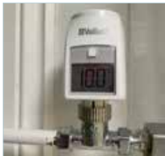
Heating controls Install smart radiator valves to control temperature in individual rooms.
