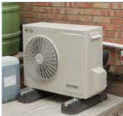
Air Source Heat Pump collect heat from the outside air and transfer it to your heating and hot water systems.
