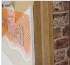
External wall insulation boards covered with a special render are applied to the outside of the house.
