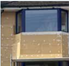
Bay window walls. Insulate either internally or externally to reduce heat loss and improve comfort levels.
