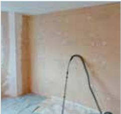
Internal insulation. Woodfibre boards are applied to the inside of external walls and covered with lime plaster.
