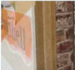
External wall insulation. Insulation boards covered with a special render are applied to the outside of the house.
