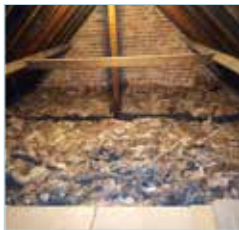
Loft insulation. Extra layers of insulation (up to 300mm) are rolled out between and over the joists.
