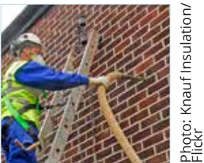
Cavity wall insulation. Polystyrene beads in resin are blown into the wall cavity through drilled holes.
